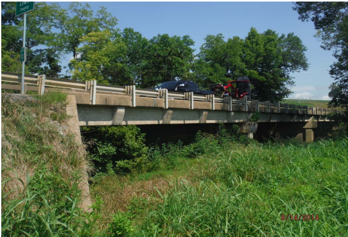
The existing bridge is a three-span RCDG structure, built in 1935.
